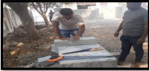
Fig: Cutting of wall
