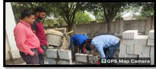
Fig: casting of wall
