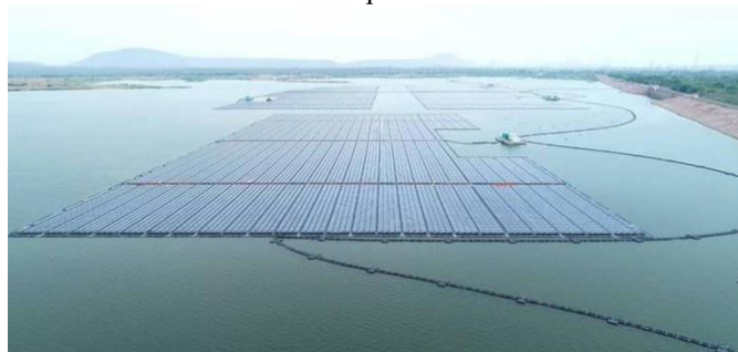
Figure 1 100 mw floating solar power plant at Ramagundam, Telangana
