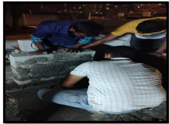
Fig: Plaster with FRP mesh
