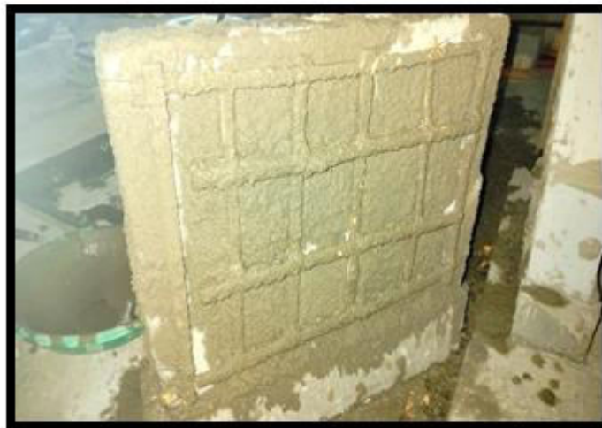
Fig : Plaster with Bamboo Fiber mesh
